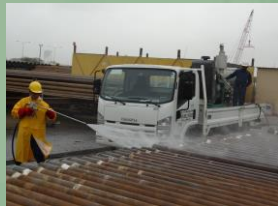
Hydro Jet Cleaning
